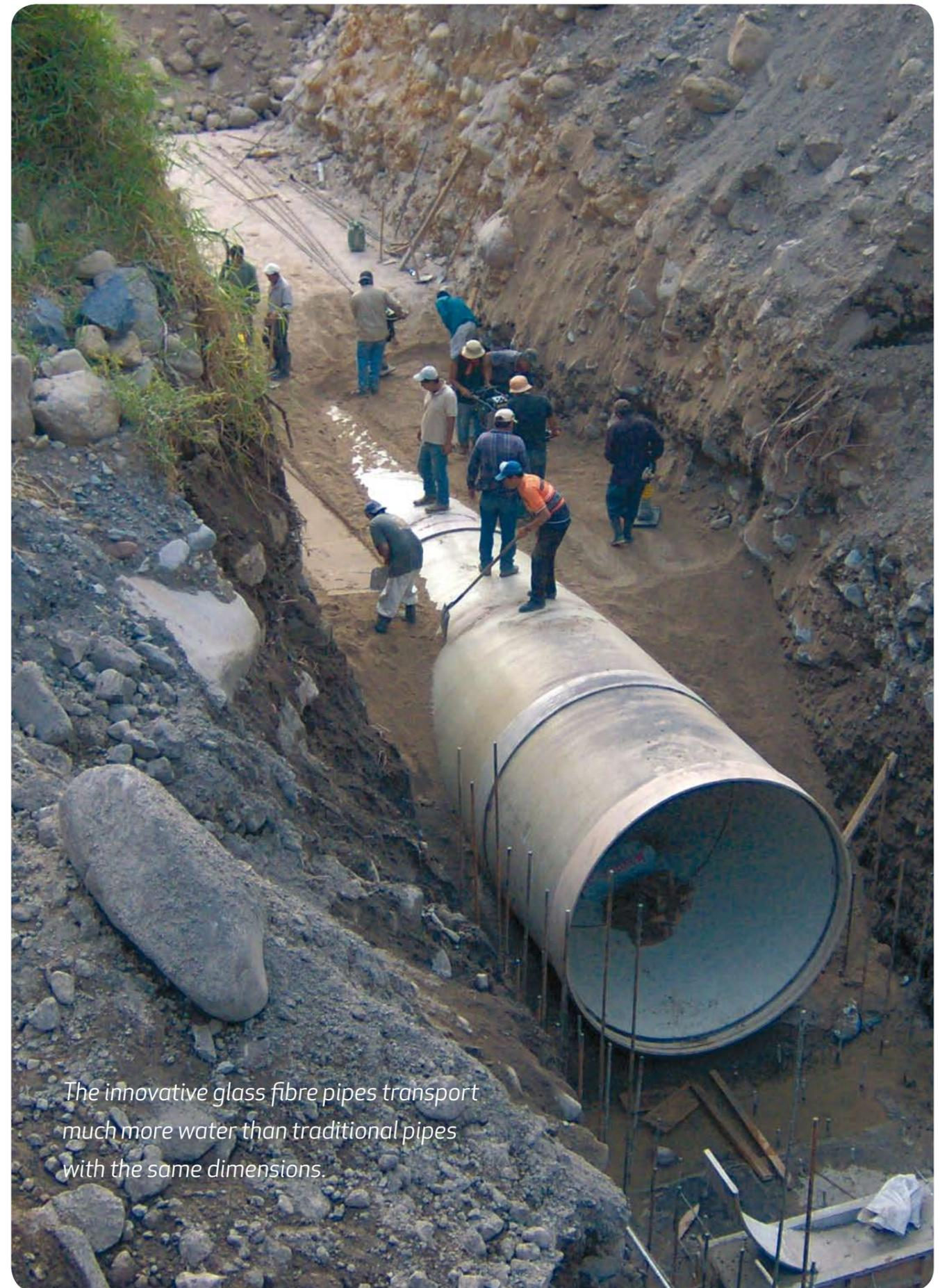
The innovative glass fibre pipes transport much more water than traditional pipes with the same dimensions.
